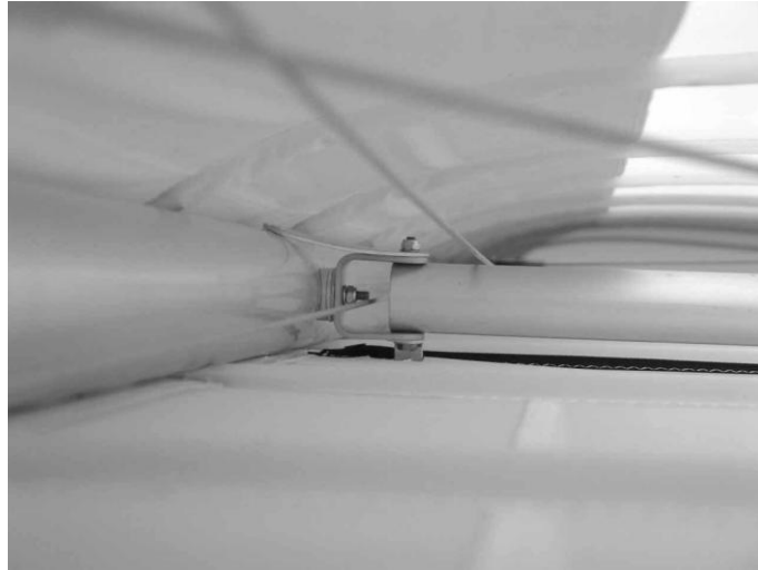
Figure 173 cable routed through U-bracket.
