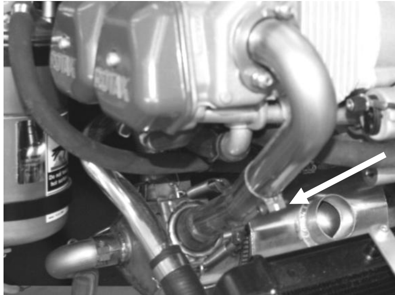
Figure 228 Port front pipe, showing clamp on sliding section
