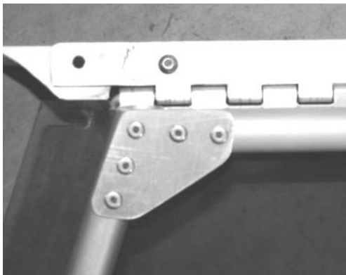
Figure 324 upper corner gusset plates.
