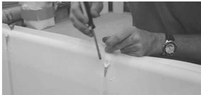
Figure 190 secure the battens in position.
